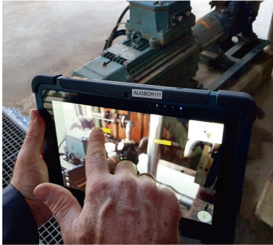
Digitally supported plant inspection using the UBIK® software from Augmensys.
