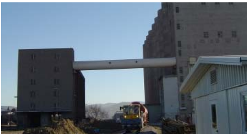
Graphic 2: Coal conveyor belts in loading and storage areas are typical installations for linear heat detection sensor cables.
